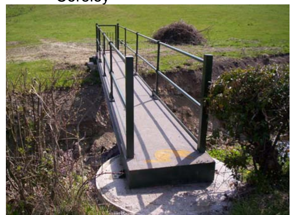
New Bridge on Minsterley BW 14
