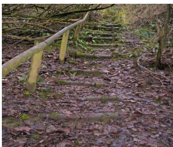
Steps requiring replacement
