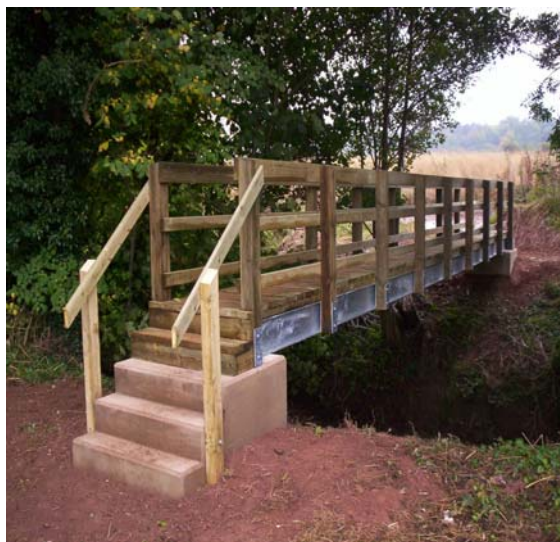
New Bridge on FP 8 Morville
