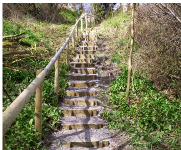
Steps replaced with the help of local P3 group
